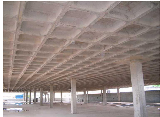
Figura 65 – Laje nervurada com moldes plásticos. ( http://www.flickr.com/photos/atex ).
